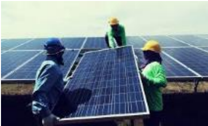
Additional 500 KW solar panel Installation
